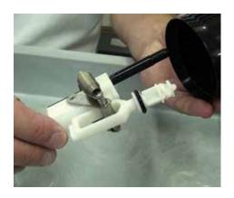
**Step 12:** Slide the actuator assembly out.
