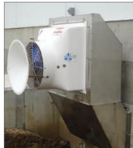
Pit transition for 24" fan mounts on pit sidewall over suggested concrete opening of 43" x 19". Reduces trash buildup in fan housing and allows use of discharge cone to increase fan delivery. Ships assembled.
