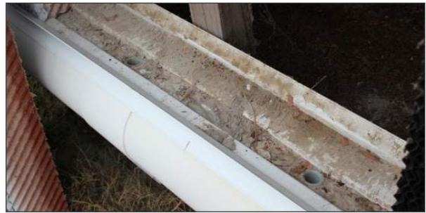
But by far the most important management practice for cool cell maintenance is to drain and replace the water often. Even with the use of chemical agents, a build up of contaminants occurs in the trough. How often to replace the water depends on water quality and the amount of the time the system operates each day. Once a month is an absolute minimum during periods of heavy use to flush grit and dirt from the system.
