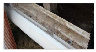
But by far the most important management practice for cool cell maintenance is to drain and replace the water often. Even with the use of chemical agents, a build up of contaminants occurs in the trough. How often to replace the water depends on water quality and the amount of the time the system operates each day. Once a month is an absolute minimum during periods of heavy use to flush grit and dirt from the system.
