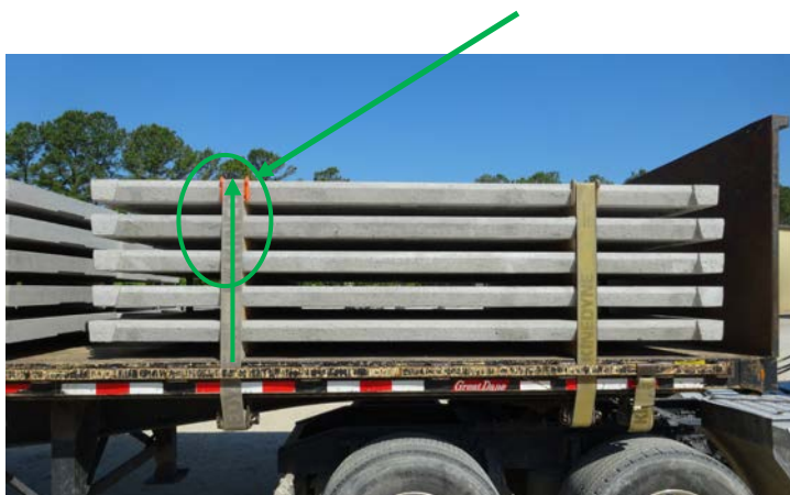
Correct tie down strap location
